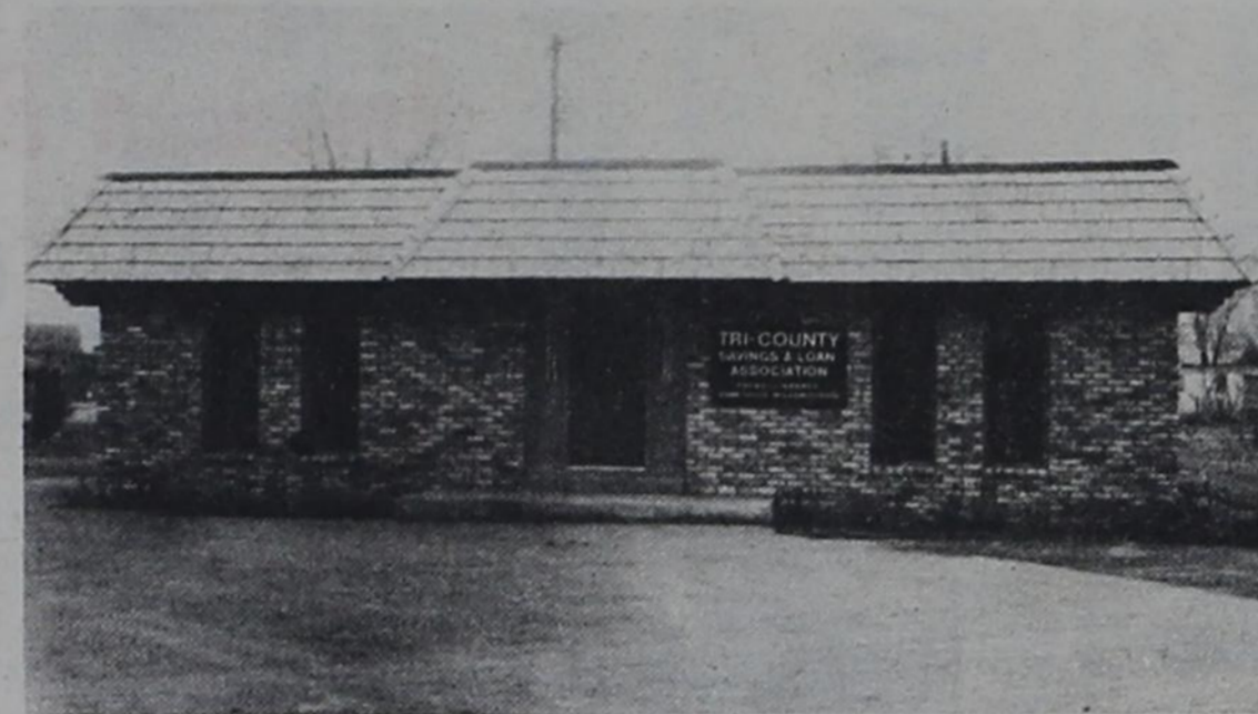
BRANCH FARWELL — Tri-County Savings and Loan Association moved into Farwell earlier this year with this new branch office at 205 Ave. D. Tri-County, which is headquartered in Muleshoe, now has branches at Farwell, Friona and Littlefield.
