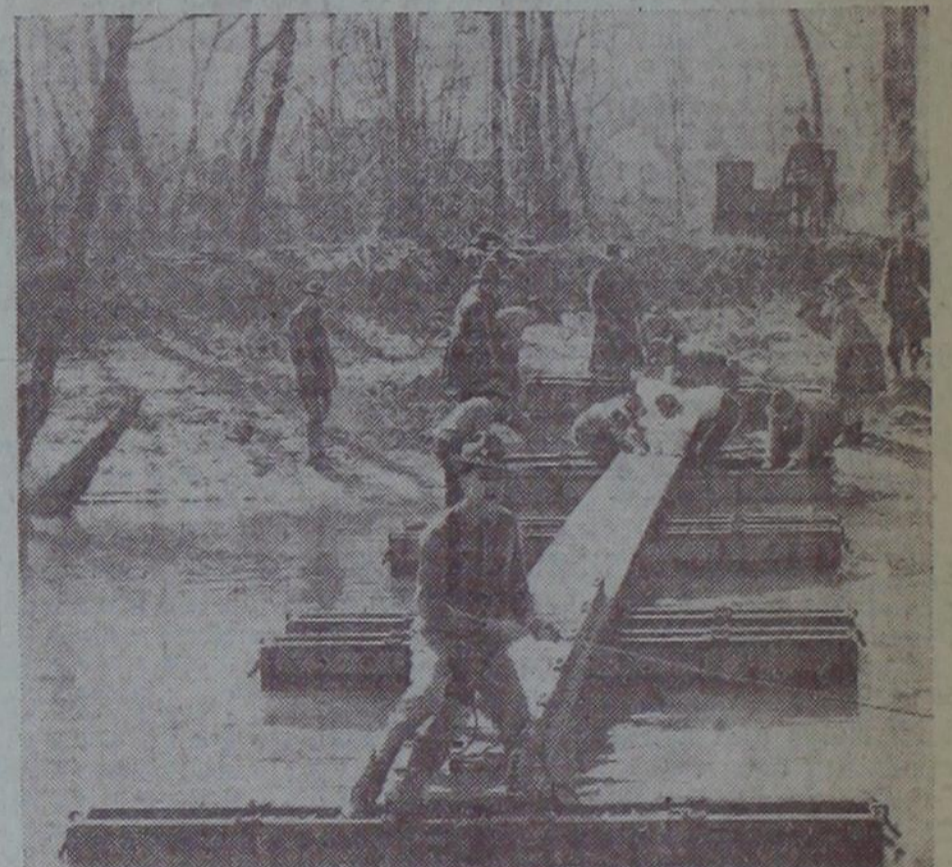
ENGINEERS BRUSH UP —Units of 121st Engineers construct 72-foot pontoon bridge across Patuxent river at Fort Meade, Md., as part of their training under U. S. defense program.
