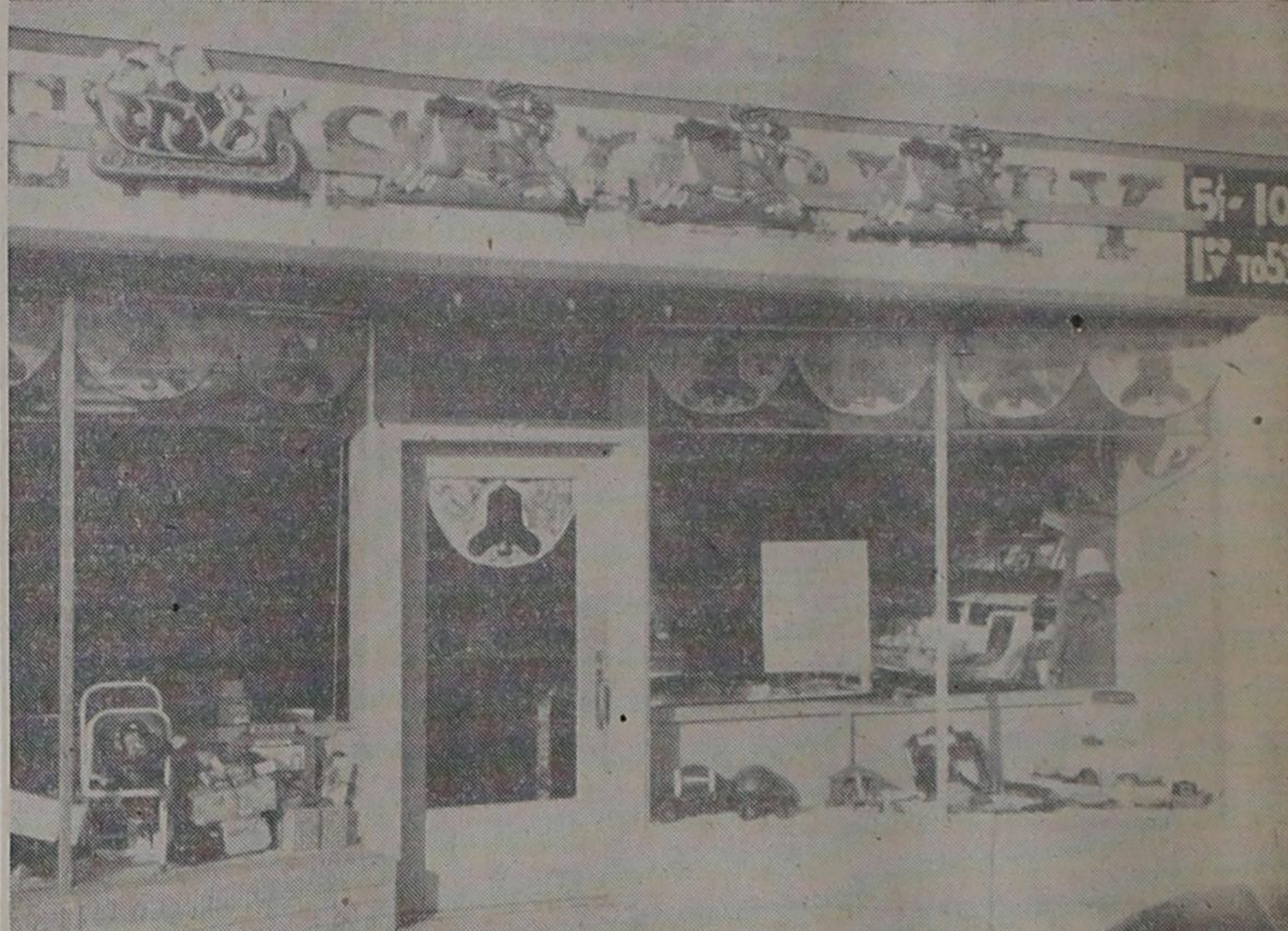
Like many other Friona businesses, Lewis Variety pleased the public this year with an attractive display of decoration tied around a Yuletide theme. Near the top of the building can be seen Jolly Old St. Nick complete with sleigh and reindeer, and bells and other decorations in the windows and door round out the motif.
