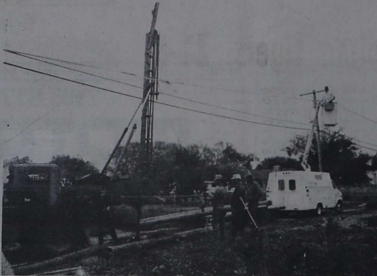
Upgrading Cable System
