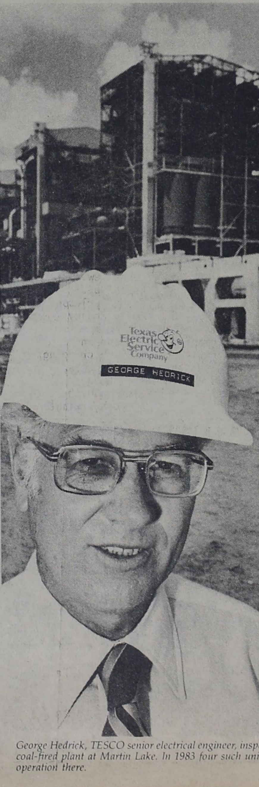
George Hedrick, TESCO senior electrical engineer, inspects a lignite coal-fired plant at Martin Lake. In 1983 four such units will be in operation there.
