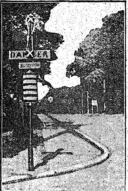
Arm at Top of Signal Post Revolves and Large Gong Sounds at Approach of Trolley Car.
