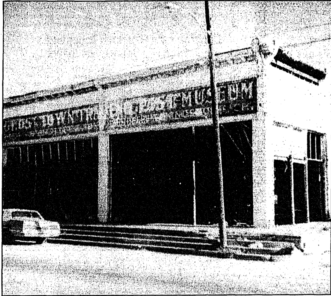
Major renovation going on at Kelley building.
