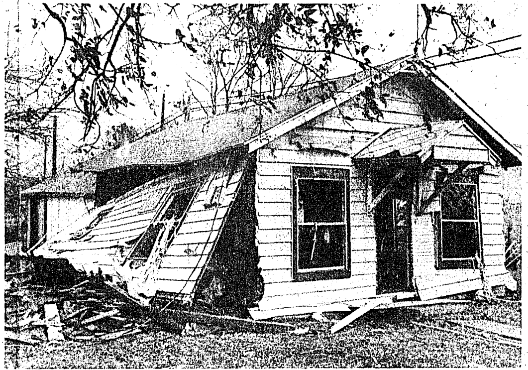
Result of Explosion ...looking from front view of house.
