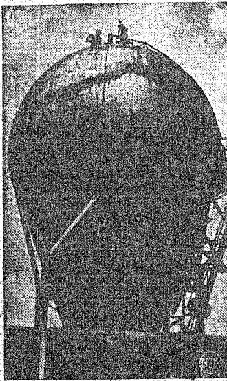
Silhouetted against the clouds, two workmen are dwarfed by the 65-foot Westinghouse atom-smasher in Pittsburgh, Pa., as they resurface the giant tank to prepare it for a research program aimed at harnessing atomic power for peacetime use.
