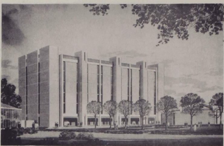
NEW BIOLOGY BUILDING - Construction has begun on the new Biology Building in the area west of the Science Building. The $3.9 million structure will be equipped with the latest facilities and should be ready for occupancy by the fall of 1969.
