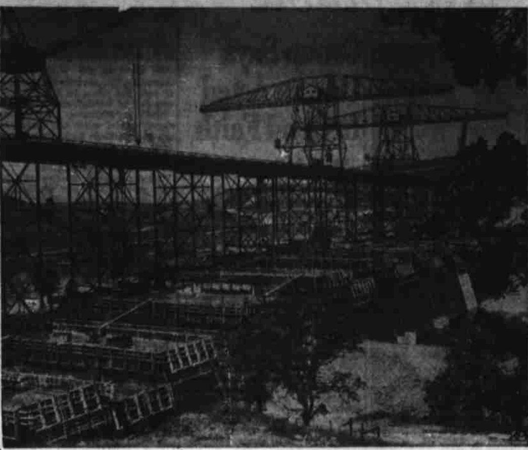
WELL UP IN THE MILLIONS —Against the surrounding hills and sky appears Grant dam in California, viewed from a point just upstream in the reservoir area. The big cranes on the long steel trestle have placed one million cubic yards of concrete, weighing twice that many tons, in the dam which is being built as part of the Central Valley project.
