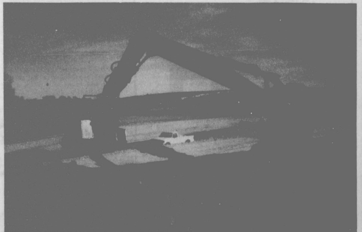
This is the large backhoe digger Central Plains Construction brought to the Palo Duro Dam site to dig the slurry trench underneath the middle of the dam. The trench was filled with a mixture that will not allow water to drain beneath it.
