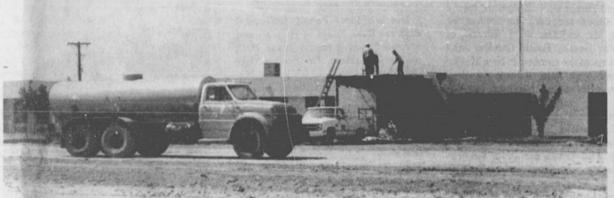
Off Comes the Roof! Workers are making progress on the new 40 bed addition to the Hansford Manor. The new addition should be completed in less than one year. The base dirt for the manor has been packed, and engineers are preparing to dig the foundations in the near future. Drive by today and watch the excellent work going on at the new manor site!
