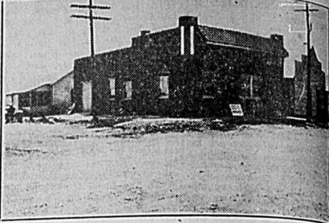
WESTERN TELEPHONE PLANT, SPEARMAN, TEXAS.
