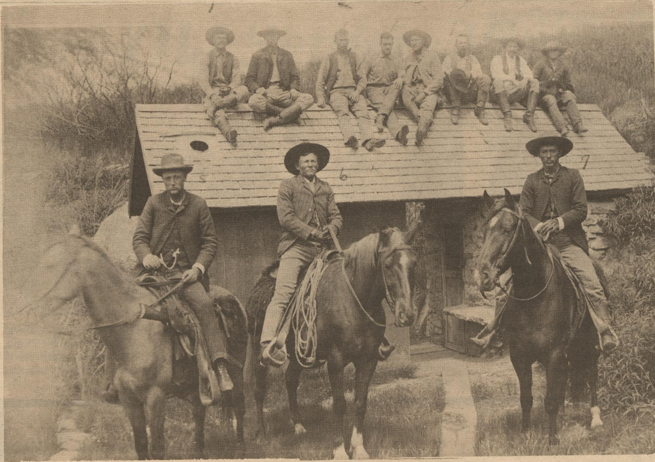
The Matador Ranch spring house below the tank dam was a two room affair with a dog trot between. The rock half-dugout on the right probably served as a cooling house with a running water trough. A handy stone ledge by the screen door was incorporated into the design. For a time, the building was a bath house for the cowboys and later served as a bakery, though by this picture the stove pipe had been removed. The known identity of the Matador cowboys numbered by Harry Campbell is as follows: On the roof, is (1) the mustashioned Joe Beckham, who later became the "outlaw sheriff"; (2) Jeff Harkey, brother to the two Harkey boys who died in separate shoot-outs at Mott Camp; (3) Bob Stelza with cartridge belt and high heeled boots; (4) Bill Wheeler, also with cartridge belt. On some very sleek, well-fed mounts are (5) Simpson, who sported a gold watch chain and carried a rifle in a scabbard; (6) Bus Baker, whose loosely coiled rope and wooly saddle bags adorned his high backed saddle; and (7) Jeff Boone, who later died of blood poisoning from a wound inflicted, some say accidentally, by the future sheriff Joe Beckham. Photo courtesy of Mr. and Mrs. Vance Campbell.
