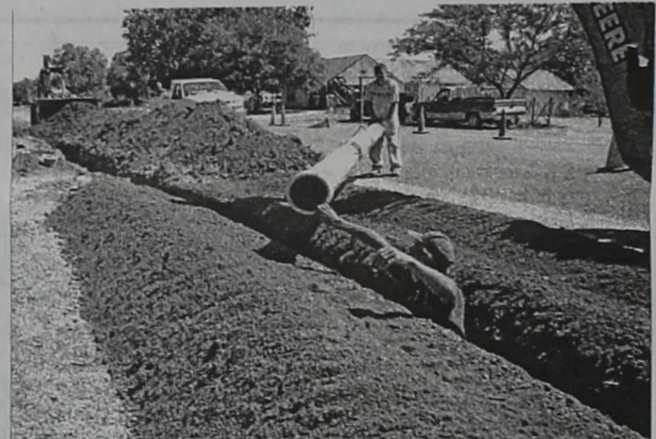
CREWS are busy replacing water lines in Matador.
