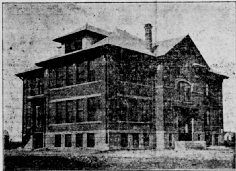
Tahoka High School Building
