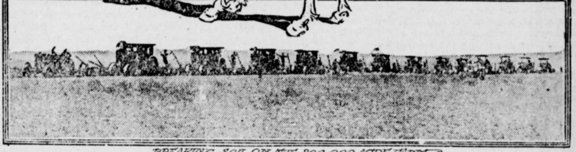
BREAKING SOIL ON THE 200,000 ACRE FARM
