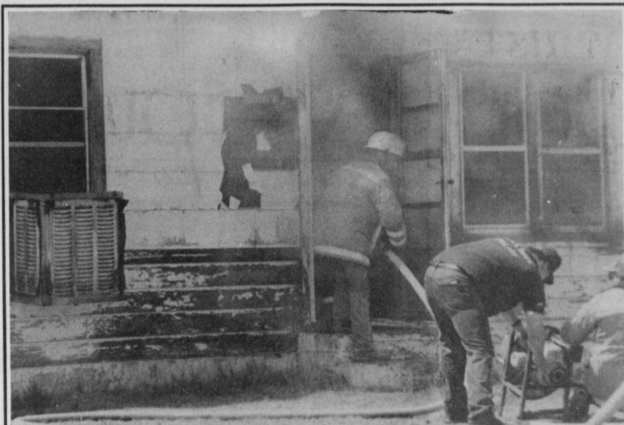
HOUSE SUSTAINS DAMAGE - Muleshoe Volunteer Firefighters worked to put out a blaze at a residence Thursday located on Highway 84 near Wilson Drilling. The home belongs to Lexie Welch and sustained about $10,000 in smoke damage, according to reports at the Bailey County Sheriff's Department.
