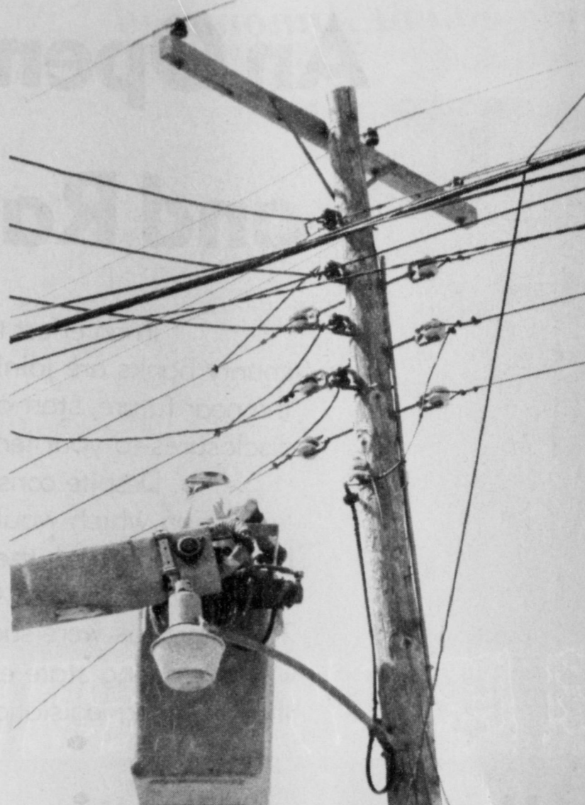
HIGH WIRE ACT. . . power company lineman Larry Whitford clips a line no longer in use from the top of a power pole.
