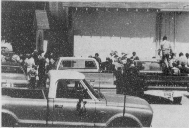
The Union Church held ground breaking ceremonies for an addition to the sanctuary Sunday, April 21 after the 11 a.m. services. The addition will increase seating capacity by one half, and will provide
