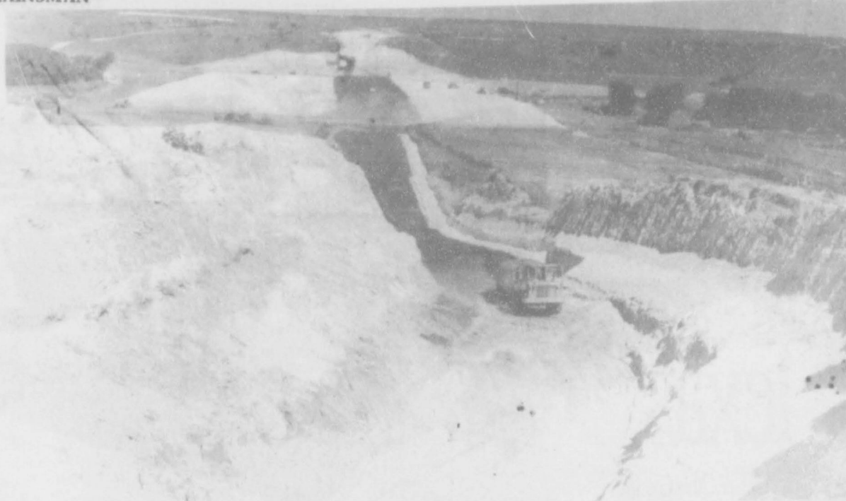
A 55,000 gallon water hauler, spraying water, moves up a trench cut in the hillside. The trench will serve to fit the Eastern end of the dam to the existing canyon.
