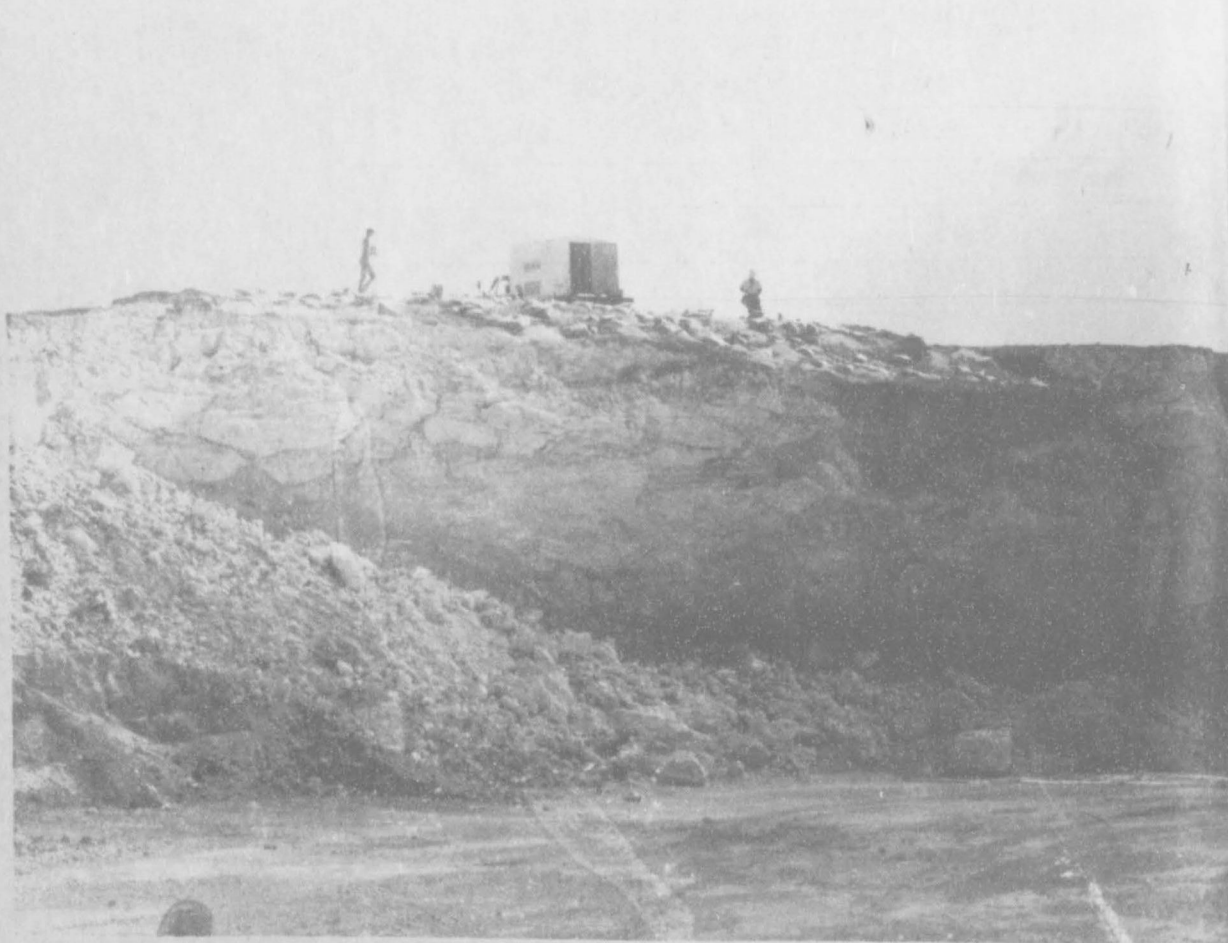
Demolition experts lay out the dynamite to be used to break away a section of rock from the edge of the emergency spillway.
