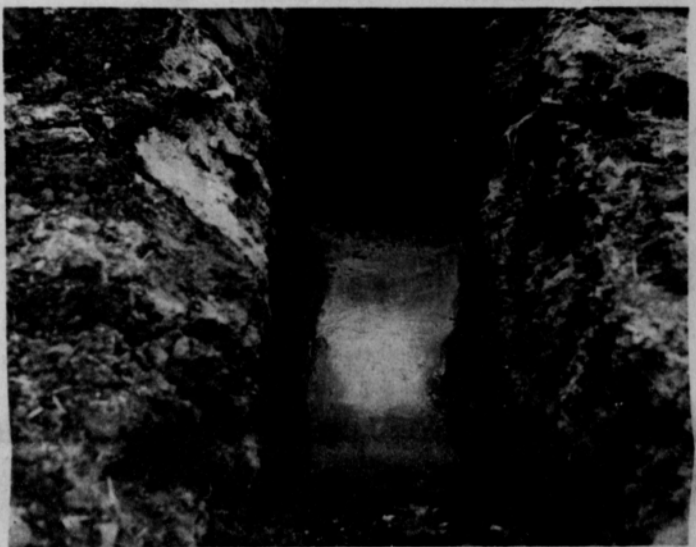
This is not a moleway. It is the opening through which an eight-inch pipe eventually will be run when work by Taylor Construction of Canyon has been completed on a new water line and installation of miscellaneous equipment to tie two new water wells into the existing system.
