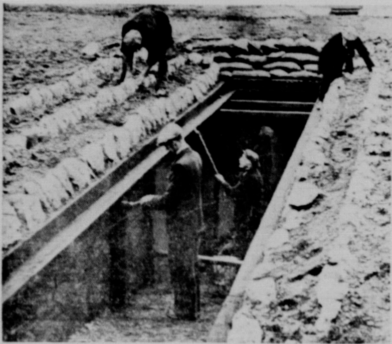
Workmen have completed one of the trenches dug on the grounds of the Imperial War museum in London during the war scare that preceded the Munich pact. Authorities will maintain the trenches as a permanent air-raid shelter in the event of future war. Safety measures of all kinds have been widely inaugurated throughout all of England as well as London.
