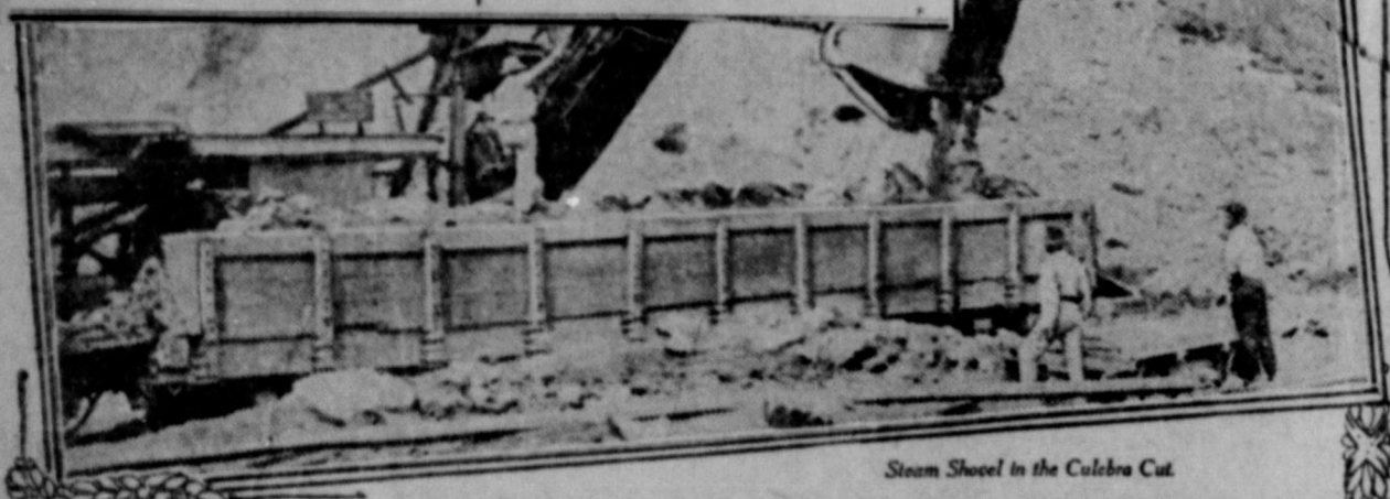
Steam Shovel in the Colobra Cut.
