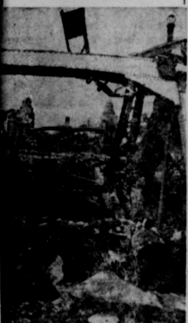
Official U. S. Navy Photo Japs' spite work. War Bonds help pay for substitute for Quezon bridge, Manila, for military movements following demolition by the enemy in historic retreat. U. S. Treasury Department
