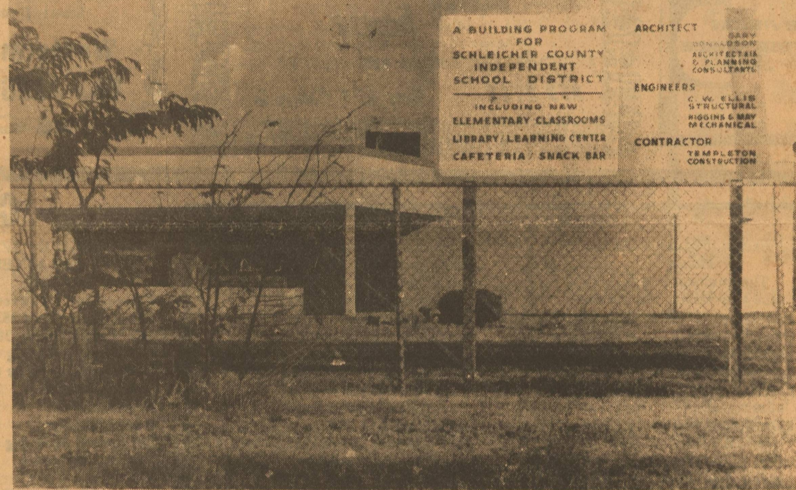
With the opening of school fast approaching, the finishing touches of the new additions at Eldorado ISD are being accelerated so that the new facility will be available for use. Shown above is the new High School Library-Learning Center.
