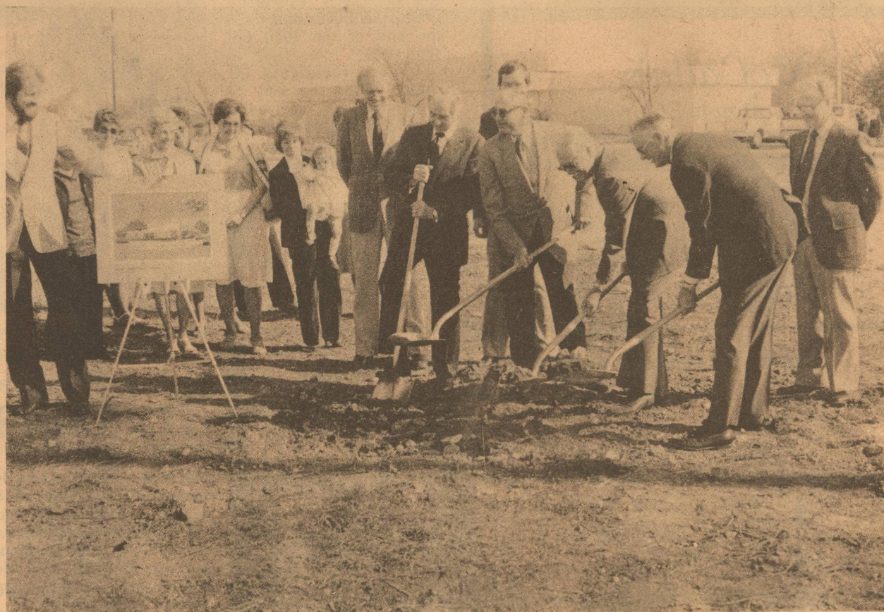
DOING THE HONORS--A small crowd watches as the directors of First National Bank turn the first shovels of dirt for the new bank building. At left is architect Gary Donaldson and building contractor Phil Templeton.
