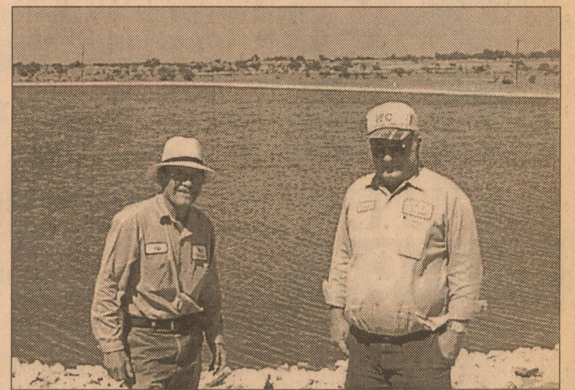
Eldorado's wastewater treatment plant is fully operational following a recent expansion project. Here, Pilo Arispe and City Superintendent Jack Dean show off the upgraded facility.
