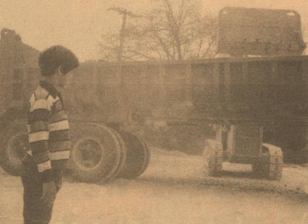
10 year old Lane Wilson gets a close-up look at the construction site of the future Mini Mart Store on highway 277 south in Eldorado. Lane is the son of Mr and Mrs H.D. Wilson of Odessa, Texas. He was a visitor in town during Easter school vacation.
