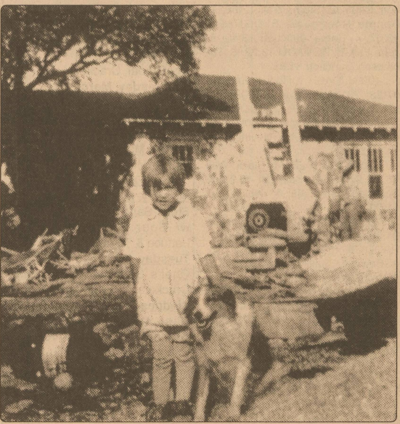
Old home place — Kathleen Crosby (St. Clair) is shown here during the construction of her grandparents rock home, under the shade of a giant oak, were the family first made its home in a tarp covered wagon after filing for and settling the land in 1901.
