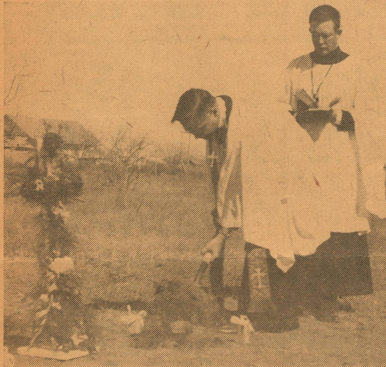
THE GROUND BREAKING WHICH TOOK PLACE IN FEBRUARY
