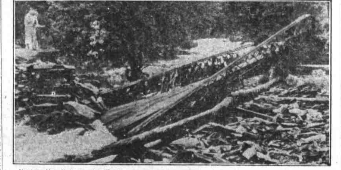
Update New York counted 37 dead, several missing and property damage amounting to several millions of dollars after a week-end of violent rain storms. This picture shows one of many small bridges washed out by torrential downpours which swept a section near Woodstock, N. Y., forcing hundreds to flee their homes. (Associated Press Photo)
