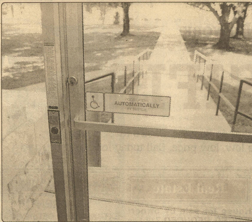
Push button access — Handicap accessibility to the Schleicher County Courthouse improved last week with the installation of this automatic door on the building's south side. Two buttons, one inside (pictured above) and one outside attached to the handrail operate the door which can also be opened and closed manually.
