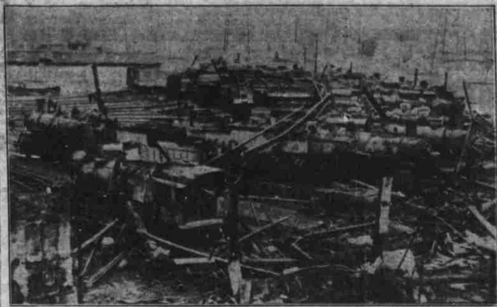
When 13 locomotive whistles blow simultaneously, it usually indicates something wrong in the railroad yards. In this case it was a $500,000 roundhouse fire in Oklahoma City. The wreckage after the blaze is shown above. (Associated Press Photo)
