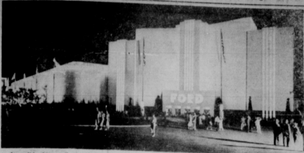
Its solid white walls flooded with many lights, the huge Ford Exposition building at the Texas Centennial in Dallas makes an attractive and imposing structure at night. Parapet lighting adds beauty to the design. The front of the building, which faces Federal Concourse, has rows of Neon tubing which contribute much to the general lighting arrangements.
