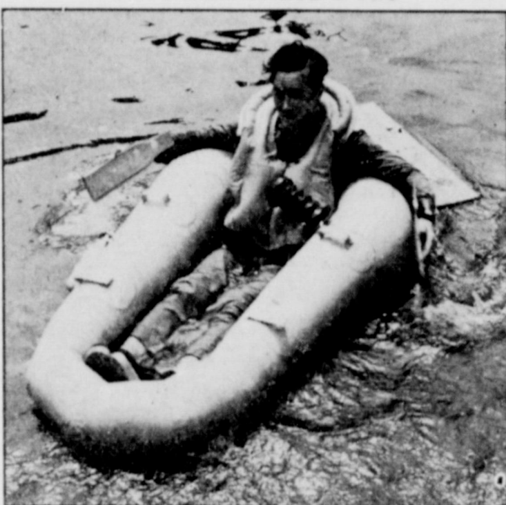
An ingenious new one-man parachute boat for emergency use on single-seater fighter planes is being tested by American armed forces. Ralph Douglas had it inflated in less than 10 seconds in a demonstration of the new life-saver. It's attached to the pilot as a seat pack.
