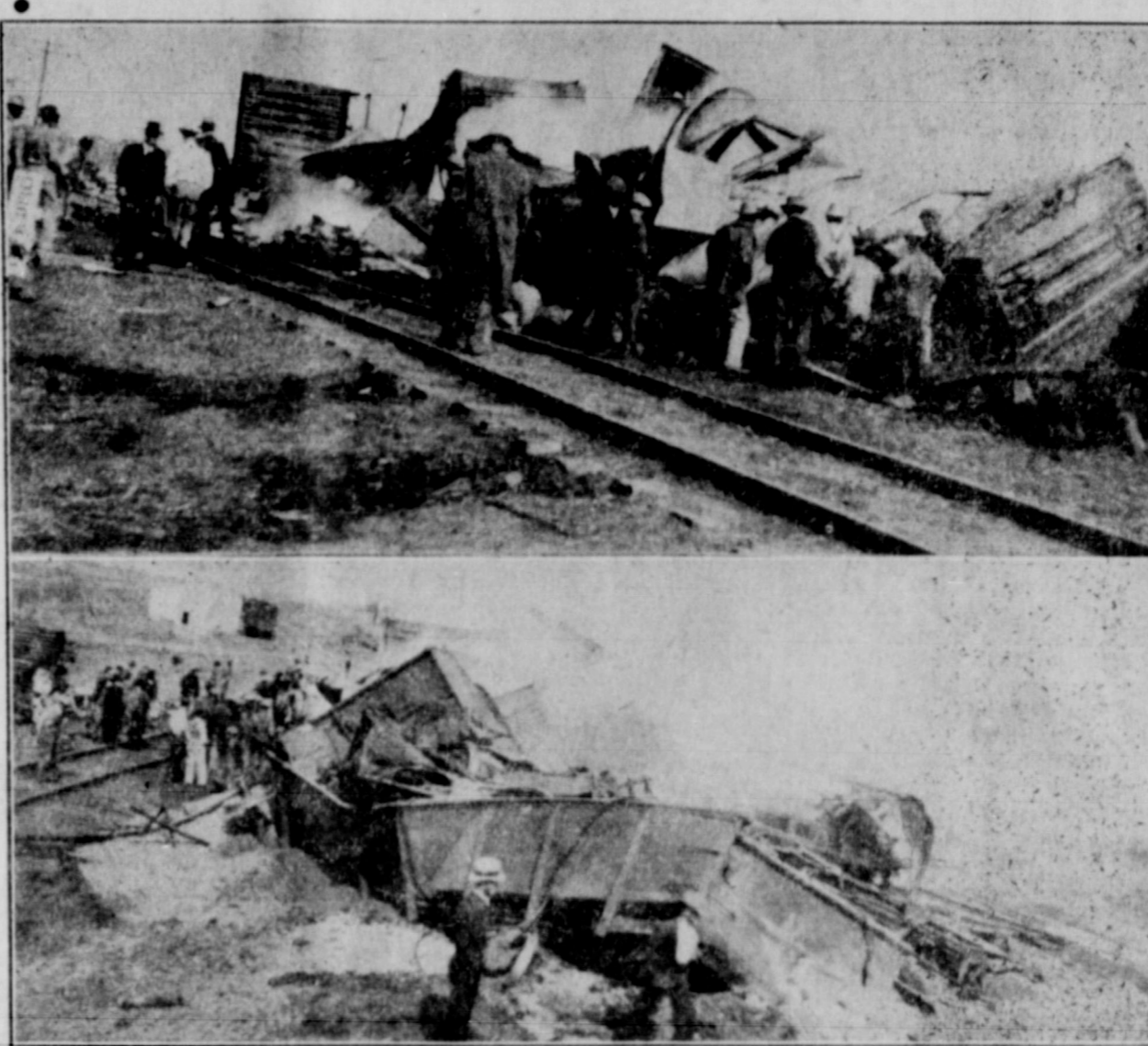
Twisted, broken steel and smouldering flames were all that was left of 16 Fort Worth and Denver freight cars when the above pictures were taken, after the cars had derailed and burned at Lelia Lake Wednesday night. Above is pictured two sections of the wreckage, showing how the cars were piled up, twisted and broken. The lower photo also shows huge piles of gravel dumped on the right-of-way. Railroad traffic was delayed between six and seven hours while the side track, at left of wreckage, was being cleared. Damages were estimated at over $16,000.
