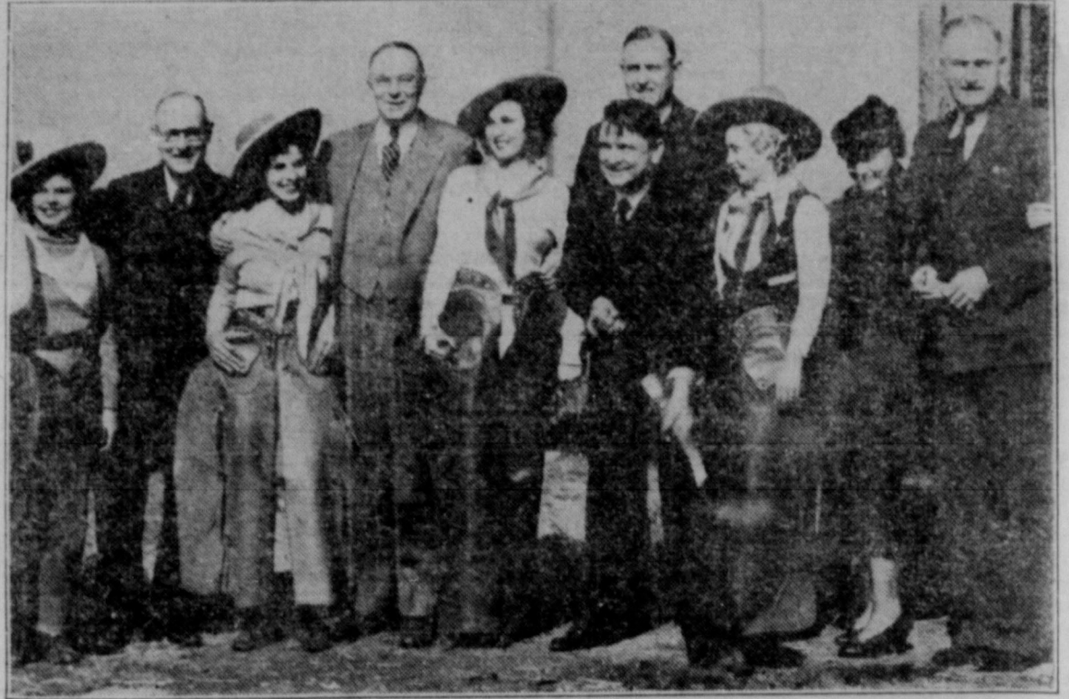
Mayor George Sergeant, of Dallas, is shown turning the first shovelful of ground for the city's $3,500,000 building program at the Texas Centennial Exposition. The seven buildings, all of uniform design, are to form the nucleus of a permanent civic cultural center and are to be completed by June 6, opening date of the Exposition. In the photograph with Mayor Sergeant and the Exposition Rangerettes are, left to right, Jim Dan Sullivan, president of the Park Board, which is supervising the city's program, Harry Gordon, George Chesnut and R. T. Shiels, members of the board.
