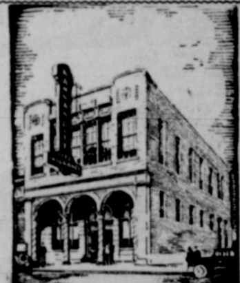
The G. S. Cummings Agency Building, Dallas
