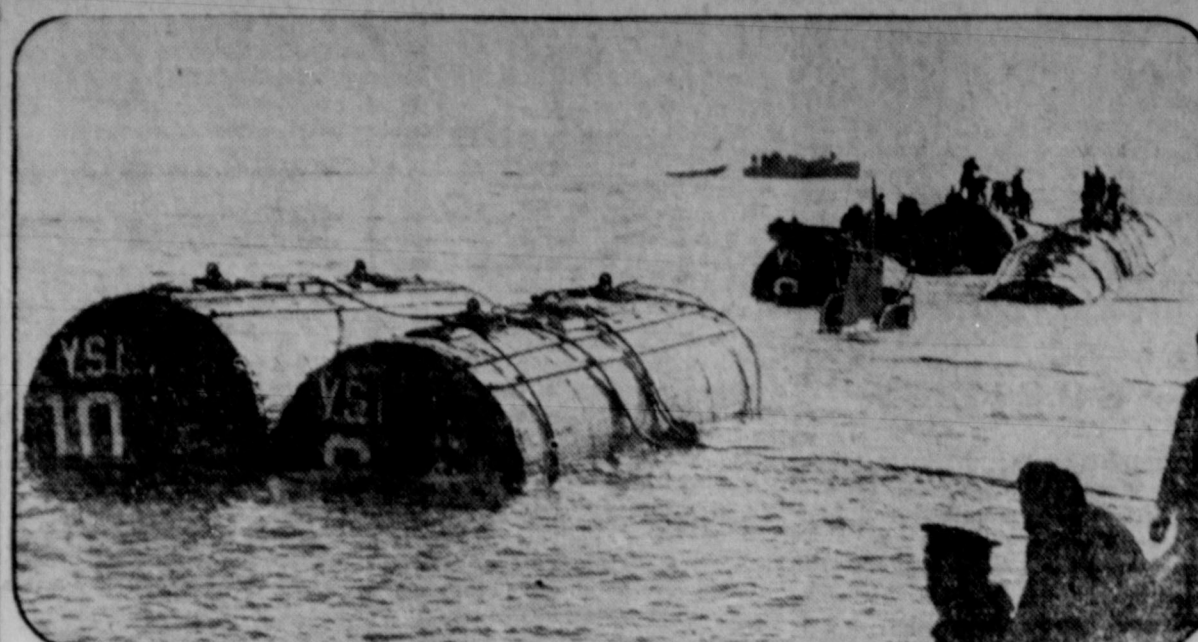
Three months after being rammed by the destroyer Paulding, off Provincetown, Mass., the ill-fated S-4 was brought to the surface, as the picture shows, by six huge air-filled pontoons and towed to the Boston navy yard. The conning of the vessel is visible between the cylindrical pontoons.
