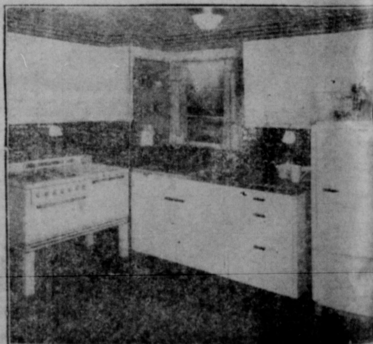
The electric range, at left, is one of the most important features of the modern all-electric kitchen.
