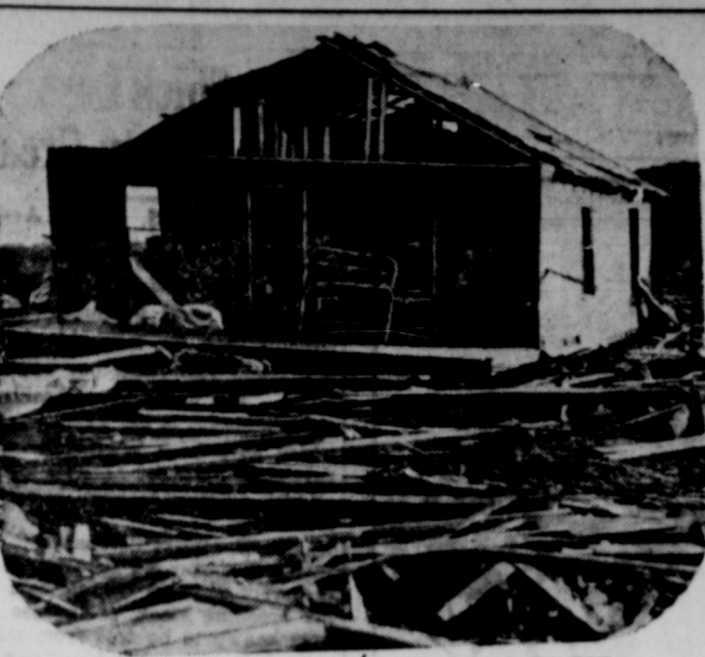
Tornado damage near Guion, Ark., showing the force of the twister that wrecked hundreds of homes and claimed more than fifty lives is pictured above. A tremendous task of relief and rehabilitation is faced in the stricken districts.
