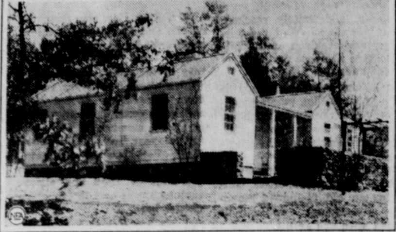
These startling contrast pictures vividly show how the standard of living has been raised for settlers in the government subsistence homestead colony at Reedsville, W. Va. Above are shown the squalid shacks in which jobless miners and their families have been living, with the polluted creek in front of them. Below is shown one of the new houses into which colonists will move, built since the program was put under way largely through enthusiastic support of Mrs. Franklin D. Roosevelt.
