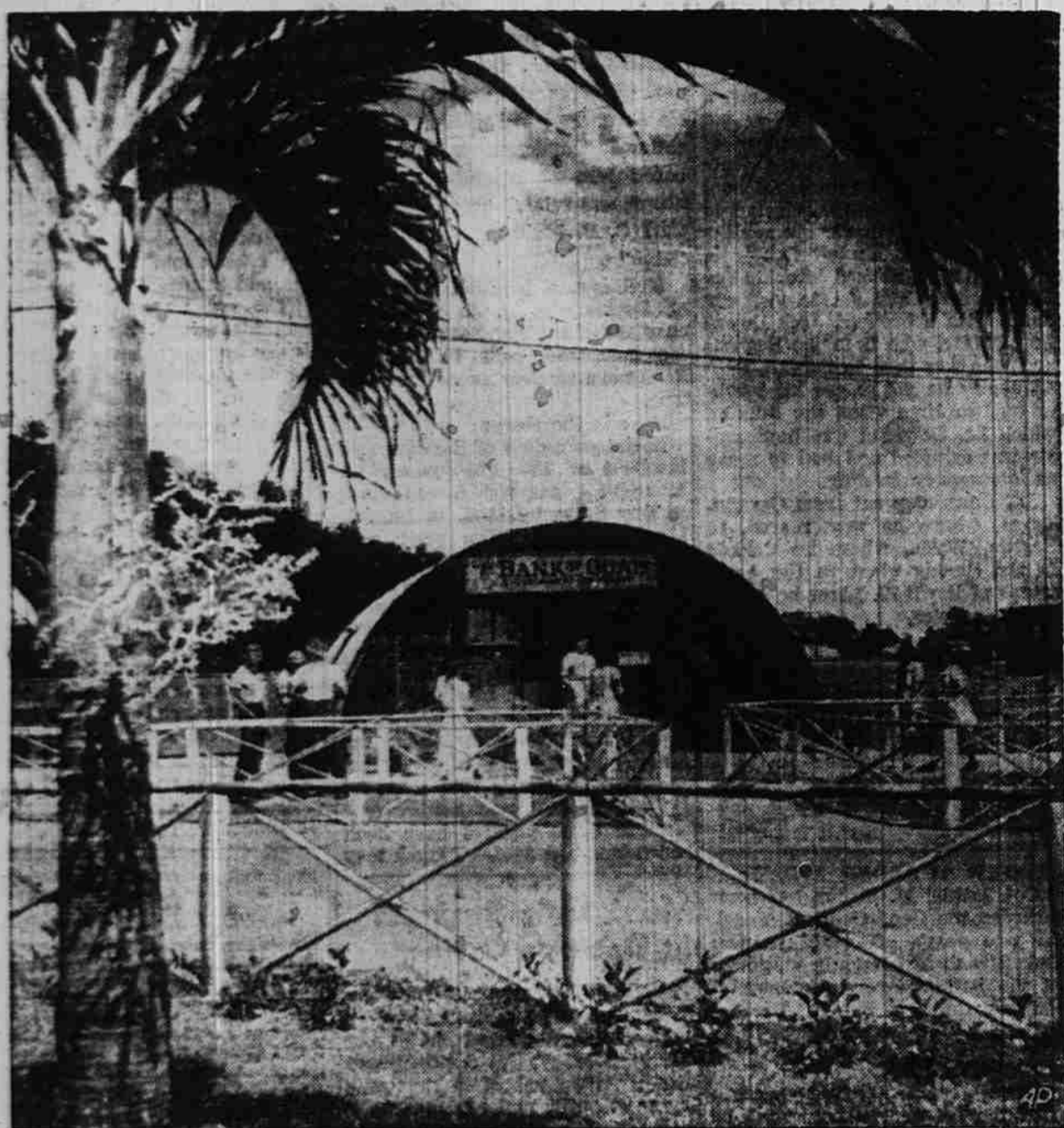
BANKING IN THE TROPICS —Housed in the ubiquitous quonset hut, the Bank of Guam cares for the flourishing community built around the big B-29 base.
