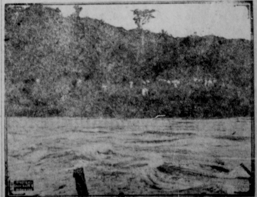
Like a mountain torrent the waters of Gatun Lake poured into Culebra Cut through the sixty-foot gap in Gamboa Dike made by the explosion of 1,600 pounds of dynamite. At Gold Hill the flood was partially dammed by the Cucaracha slide and within an hour and a half the cut was filled to lake level.
