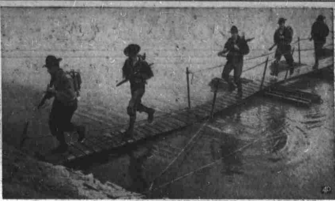
A 140-FOOT BRIDGE IN 8 MINUTES! That's the record made by 47 men who built this pontoon span across the Chesapeake and Delaware canal near Fort du Font, Del. Lieut. Thomas B. Simpson of Tuscaloosa, Ala., directed the builders, who belonged to C company of U. S. army's 1st engineers. Twenty empty one-gallon cans buoy up each float.
