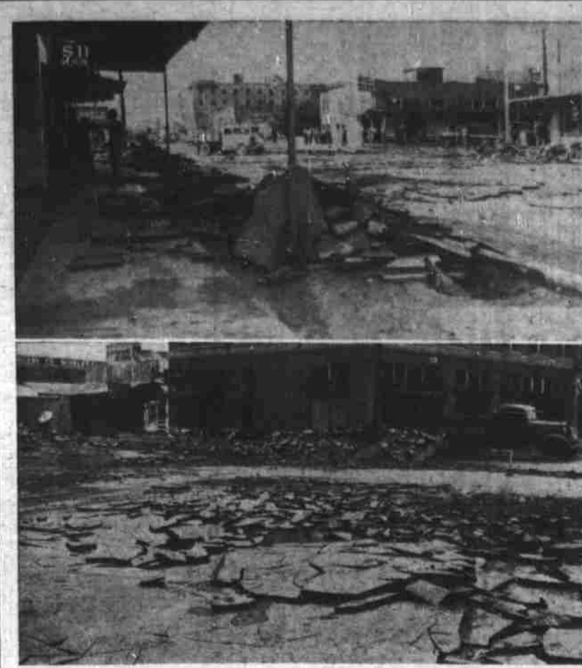
Water erosion of a devastating nature is shown in the above photo, snapped on Big Spring streets Sunday morning after the Saturday night deluge. Upper left view looks up Runnels street from near First, showing how great blocks of topping were torn up by the swift water and hurled against posts and across sidewalks. One of the larger pieces of "drift" pavement is pictured in the upper right photo. A good idea of how the force of the water
