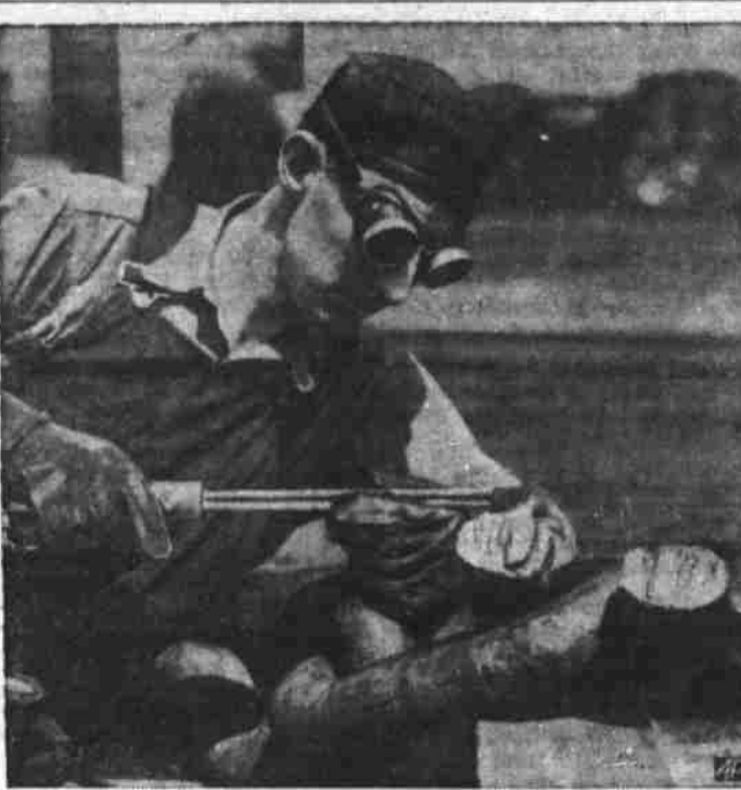
A LOOK AT LINKS —Five tons of chain with 2 1/4-inch-thick links (shown) will attach to pontoons in Squalus salvage.
