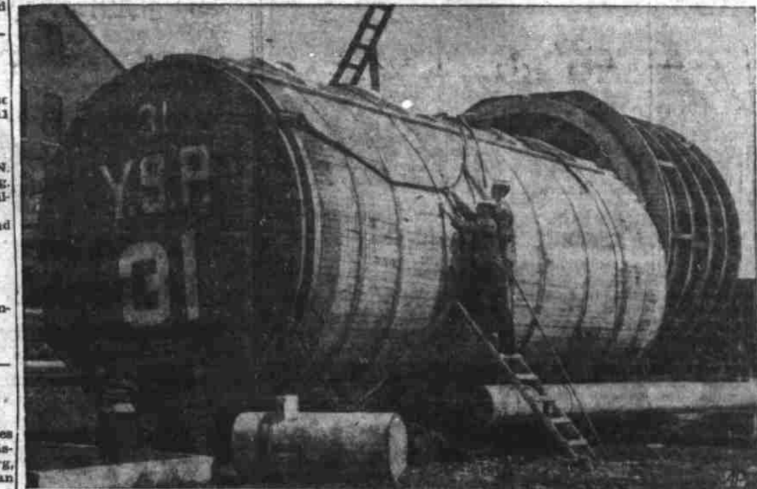
READY FOR LIFTING JOB —Workmen adjust one of the steel, oak-covered pontoons to be used in lifting the Squalus, the submarine which sank May 25 off Portsmouth, N. H.
