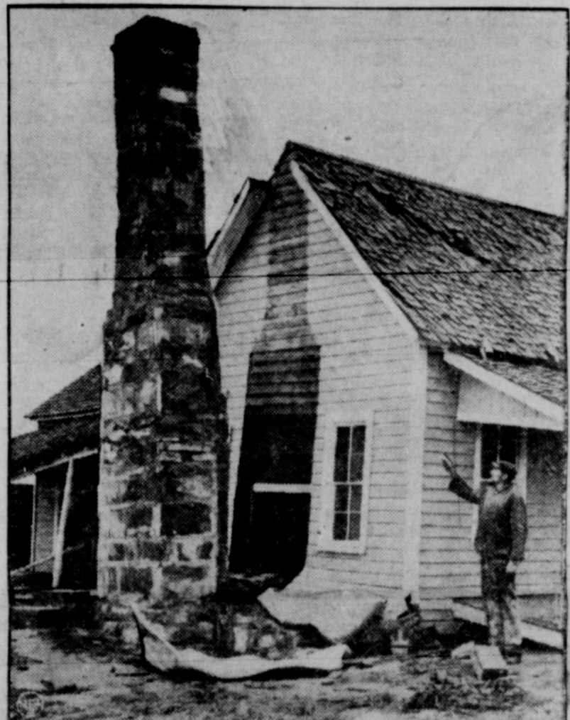
Fire still smoldered in the chimney of E. Freeman's house at Fyffe, Ala., after a tornado had moved the dwelling 15 feet and left it sagging, but still upright, as shown here. The midwinter twister, accompanied by bitter cold, killed four in Alabama and 13 in the vicinity of the Georgia-Alabama-Florida state lines, and caused heavy property damage.
